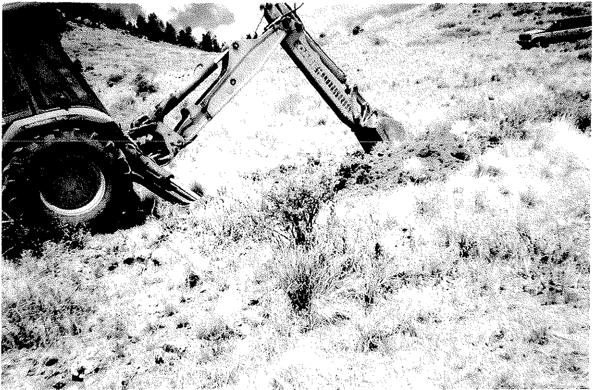
Figure 20. F7 Backhoe starting T2S Trench in thin alluvium . View -> N30°W towards T1S. Note jasper-chalcedony float over vein at backhoe wheel.
